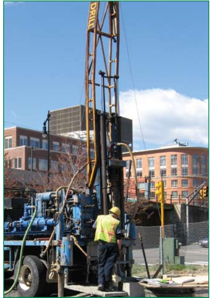
A truck-mounted boring rig performs borings for the proposed Lechmere viaduct.
