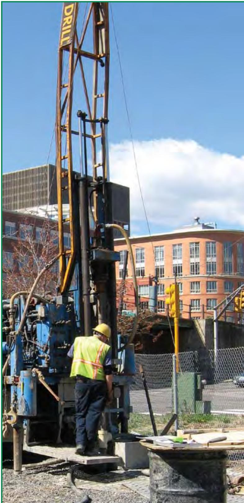
*A truck-mounted boring rig performs borings for the proposed Lechmere viaduct.*
